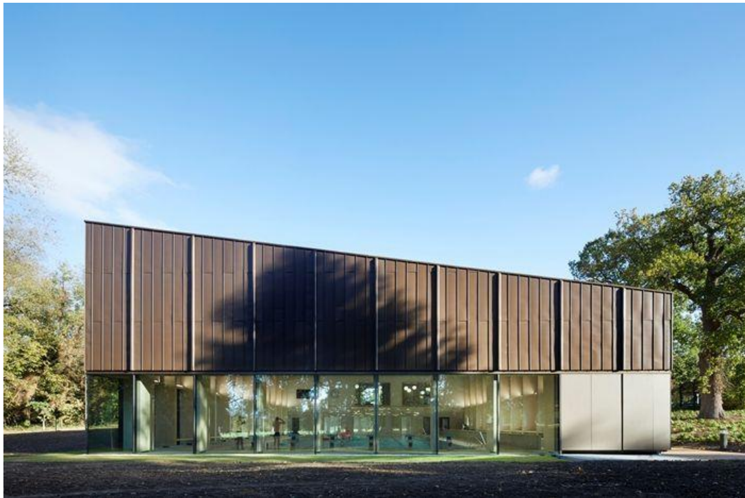
City of London Freeman's School, Swimming Pool, Ashtead. Credit: Jack Hobhouse
