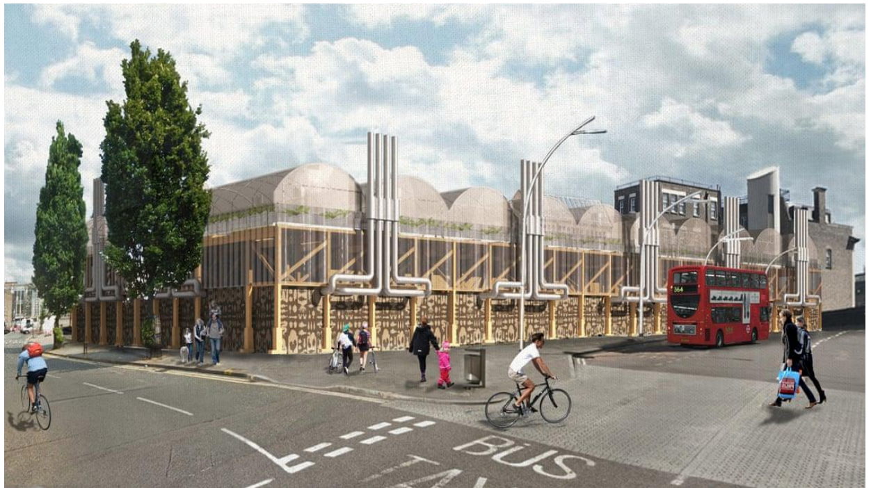
Ilford community market in east London, opening next year, will have no concrete foundations and a timber structure stabilised by rocks in metal cages. Photograph: Interrobang Architecture and Engineering
