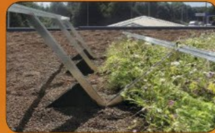
SUBSTRATE AND SPECIFIED VEGETATION
