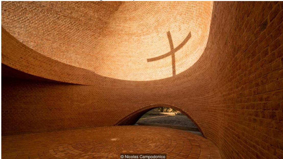
The Capilla San Bernardo in Argentina is made of salvaged farmhouse bricks (Credit: Nicolas Campodonico)
