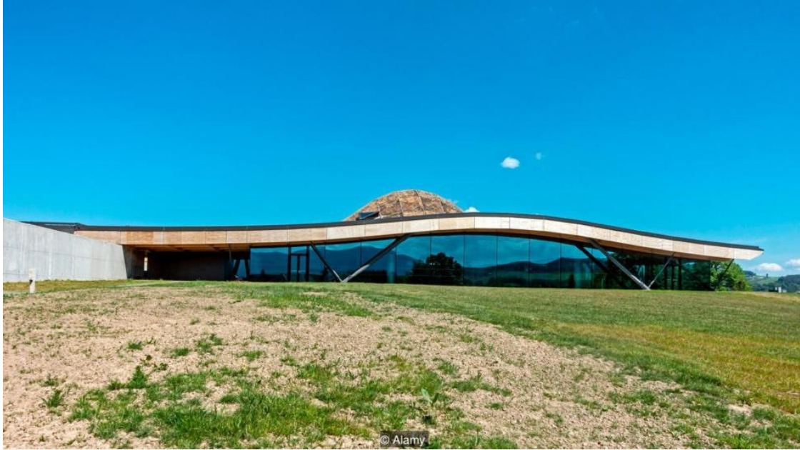
The Macallan whisky distillery has an undulating timber roof and blends in with the landscape (Credit: Alamy)
