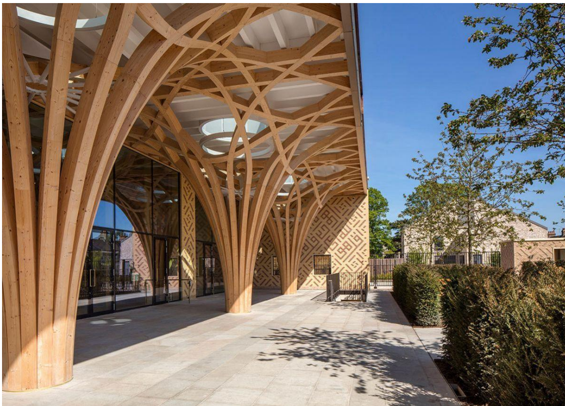
A colonnade of structural timber columns supports a portico which is the first experience of the building from the street. Credit: Morley von Sternberg
