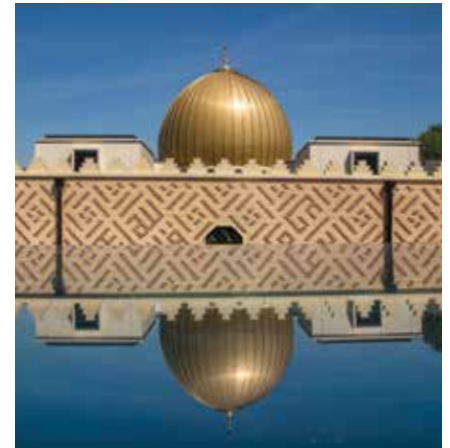
» The mosque’s dome and ventilation boxes reflected by PVs
