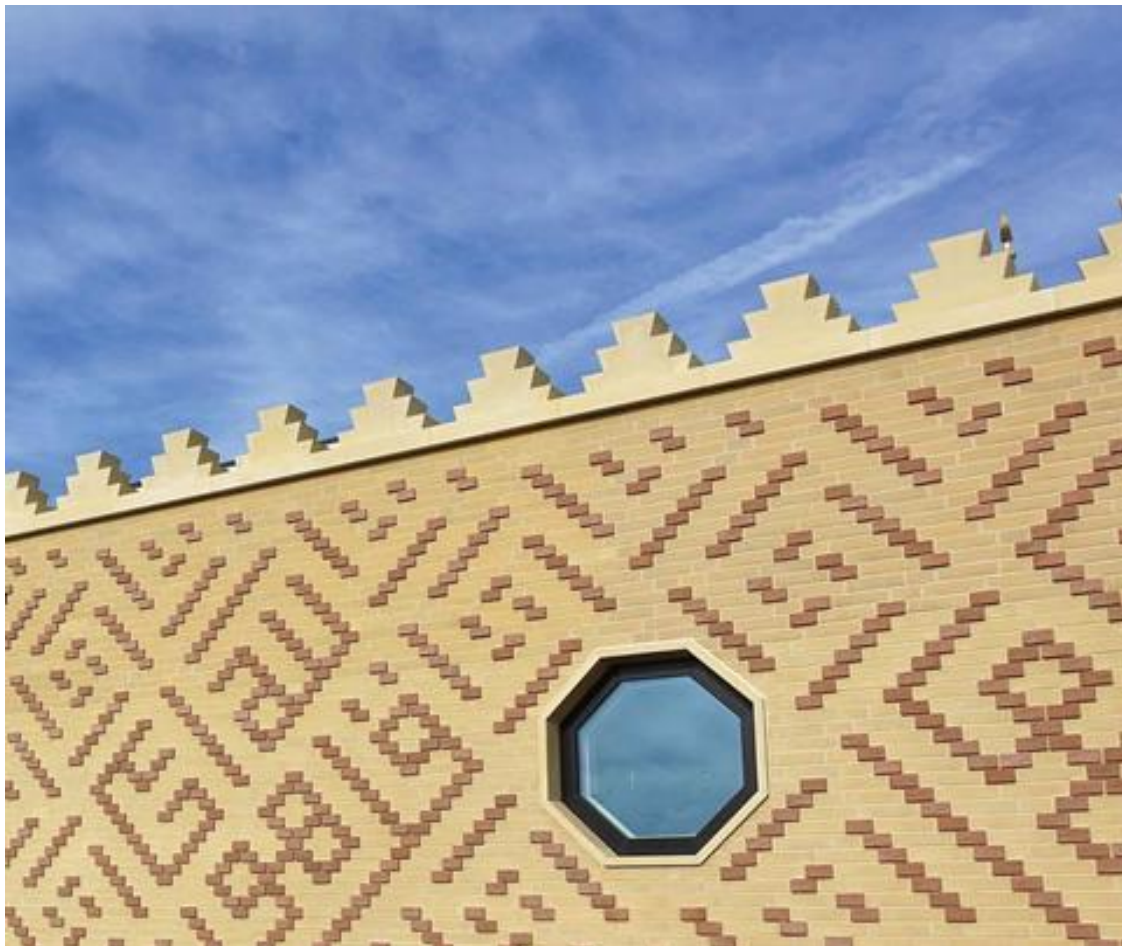
External brickwork comprises mathematical tiles and features a geometric pattern based on rotational symmetry which spells the word ‘Allah’
