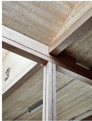
CLOCKWISE FROM FAR LEFT, A SPECTACULAR SERIES OF 16 ROOF LIGHTS SET AT 40-DEGREE ANGLES FUNNELS IN SOFT, NORTH LIGHT; THE BEECH LAMINATE-VENEER LUMBER ENABLES BEAMS AND COLUMNS TO HAVE SMALLER CROSS-SECTIONS THAN SOFTWOOD GLULAM, PROVIDING THE STRUCTURE WITH A LIGHTER AND MORE ELEGANT APPEARANCE; ARCHITECT AND CHIEF ADVISOR MARTIN FRANCIS
